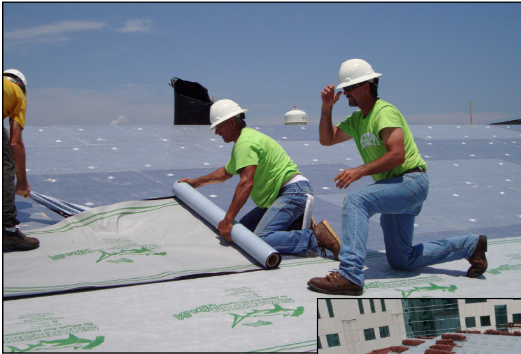
LEFT, WORKERS ROLL OUT SHARKSKIN UNDERLAYMENT AT THE KEESLER AIR FORCE BASE, BILOXI, MISS. BELOW, AN OVERVIEW OF THE HERMAN MEMORIAL HOSPITAL PROJECT IN HOUSTON, TEXAS.
